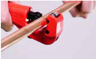
1. Cut the tube to length
