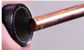
2. Deburr and remove all external sharp edges
