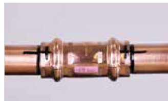
3. Mark the completed joint
