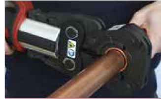
3. Complete the joint with the press tool
